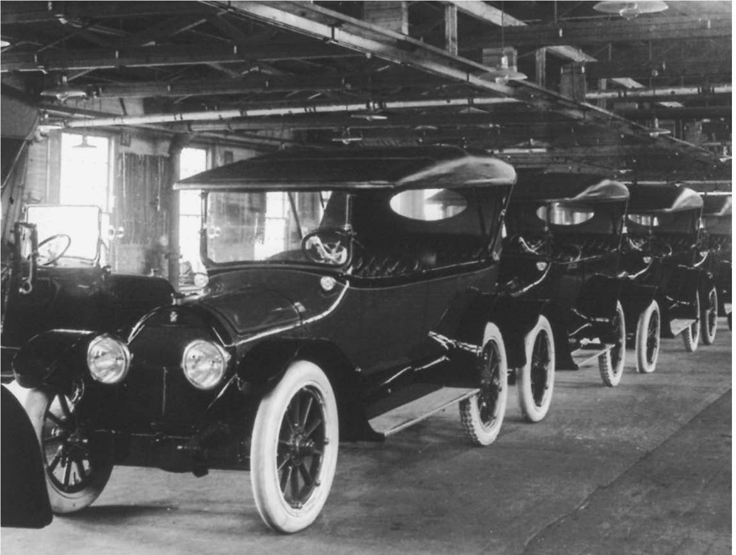
A row of completed “Tim Lizzies,” or Model T automobiles, comes off the Ford assembly line in Detroit, Michigan, in 1917. Henry Ford’s mass-production techniques brought about a revolution in transportation.
